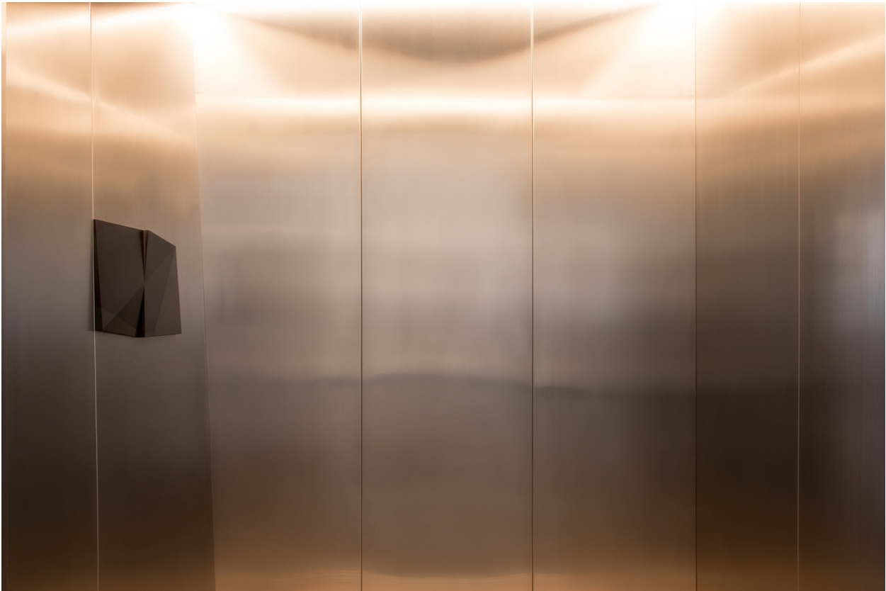
Elevator C – The left wall has two panels, and the central wall has three panels on top of the original wall of the same material and dimensions.
